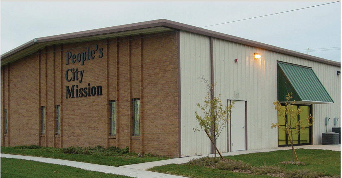
People's City Mission Homeless Intervention Center, Lincoln, NE
